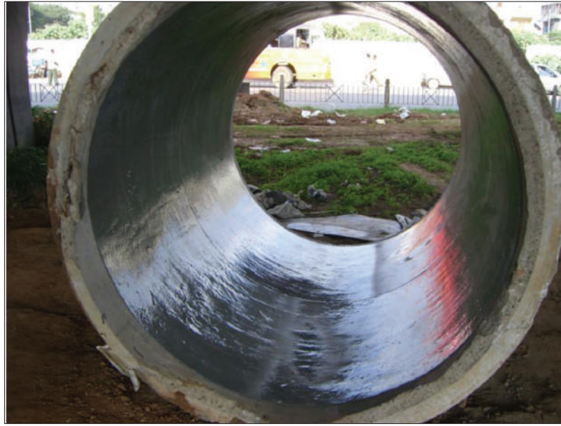
Figure 3.59 RCC Sewer pipe with protective coating
