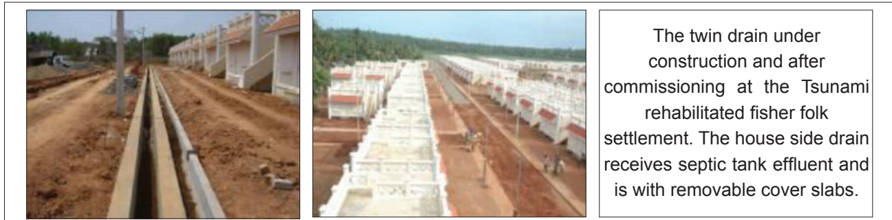
Figure 3.11 Twin drain system
