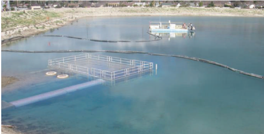
Figure 7.14 Purified water from the GWRS is piped to OCWD's percolation ponds in Anaheim, California
